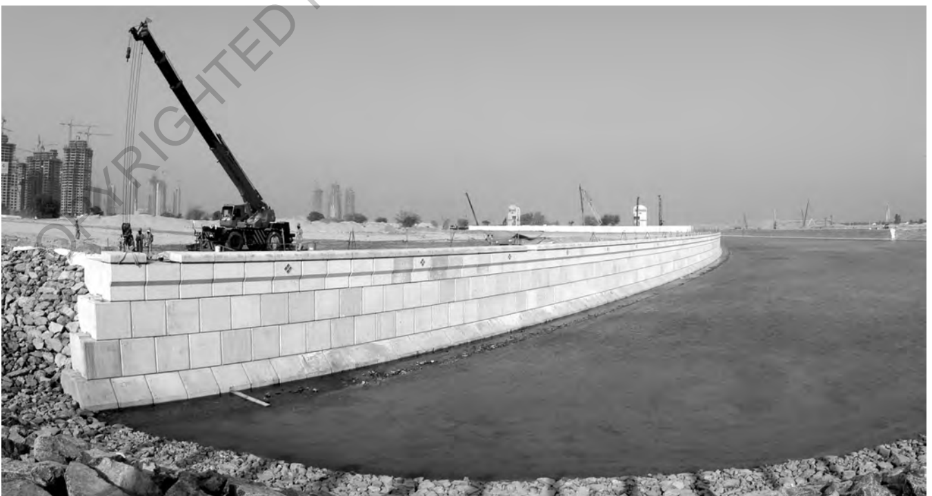
Figure 2.3 Sea wall construction with bonded blockwork. (Photograph courtesy of Abdul Rahim)
