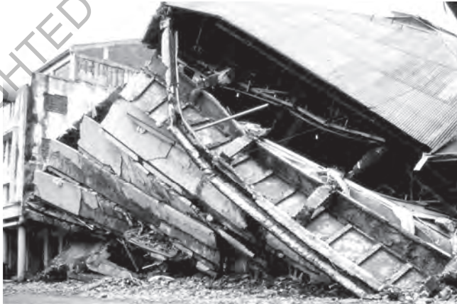
Figure 8.6 Total collapse of a multi-storey reinforced concrete building in Baguio, Philippines, 1990. (© E. Booth)
