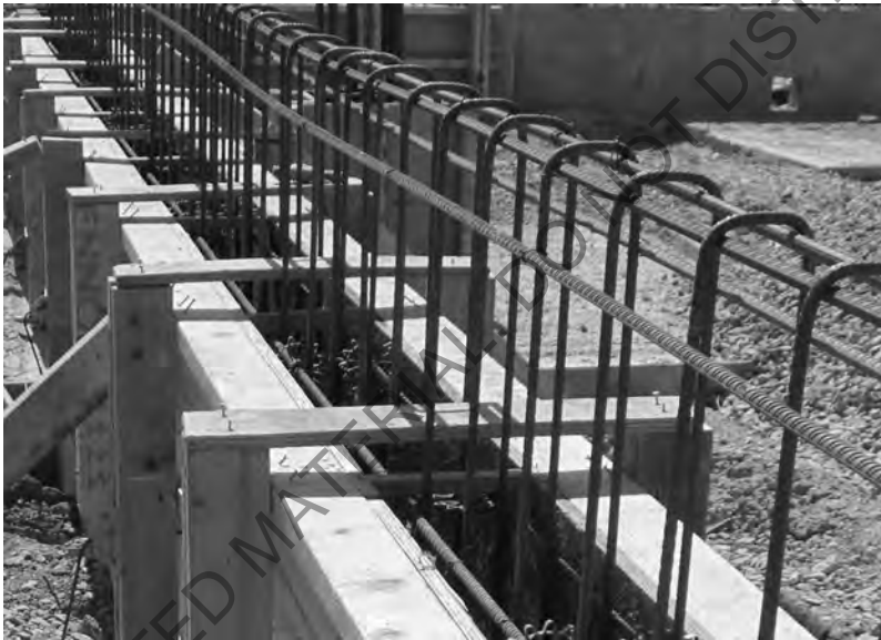
Figure 4.5 Shear reinforcement in the form of vertical links
