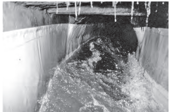
Fig. 18.13 Exposed composite geomembranes to resist high water velocities and turbulence
