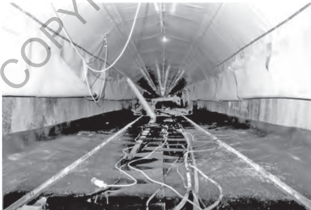
Figure 18.11 Placing of the composite geomembrane inside a pressure tunnel in the Czech Republic
