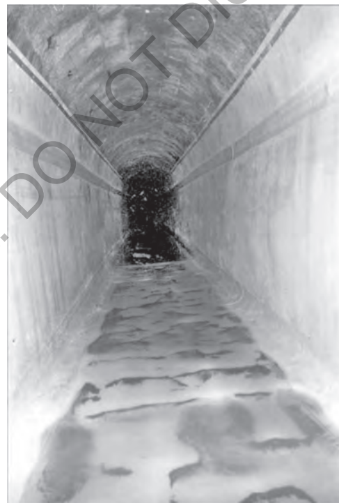
Fig. 18.13 Exposed composite geomembranes to resist high water velocities and turbulence
